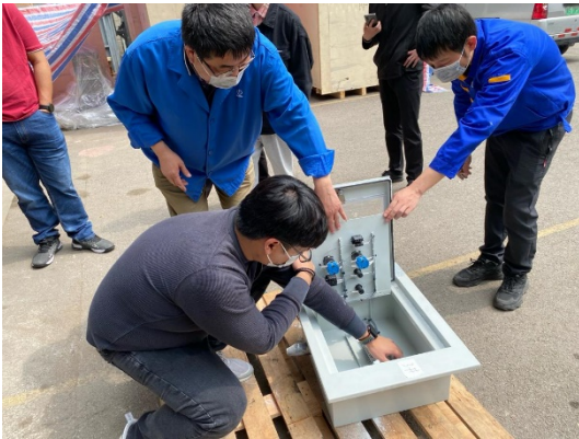
Learning from the experts... One of Sarawak Metro's apprentices inspecting a control panel under the watchful eyes of expert engineers during an attachment in China
